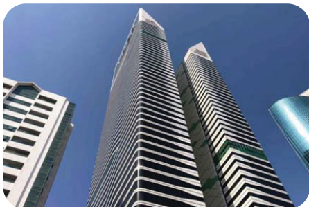
Nassima Tower, Dubai
