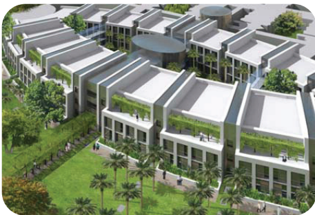
Al Wasl Maternity Hospital, Dubai
